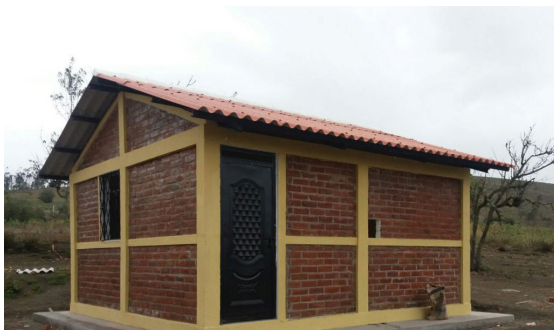
Figure 4: SDC's training house
