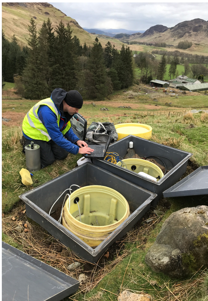
Figure 2: Maintenance of a Permanent BGS station In Scotland, with the inspection hatches of both sensor pits open. The primary sensor has been removed from its pit and is visible to the left of the person.
